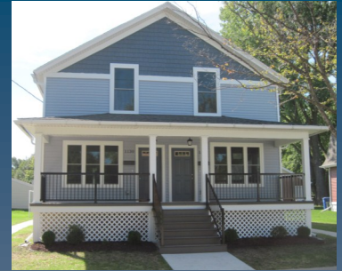
1128-1130 Day Street, two of more than 25 units renovated by NeighborWorks Green Bay in 2013.
